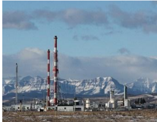
Constructing Cochrane, AB CANADA
