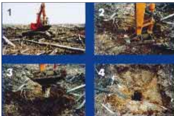
Figure 1. (Clockwise) (1) Excavator with punch attachment, (2) compacting, and (3, 4) preparing a planting hole-in-hole (courtesy of PT Group Plantations, Indonesia).
