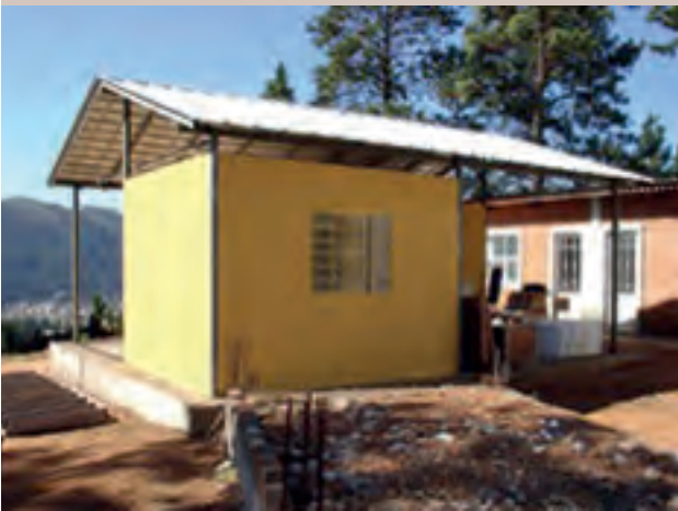
An experimental house in Brazil constructed using PG panels.
