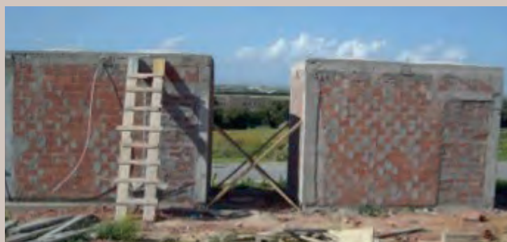
Rooms under construction sealed for radon measurements.
