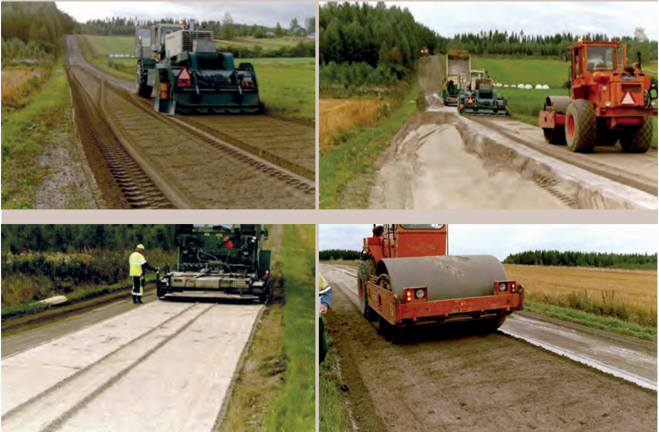
Road construction in four principal stages, Finland.
