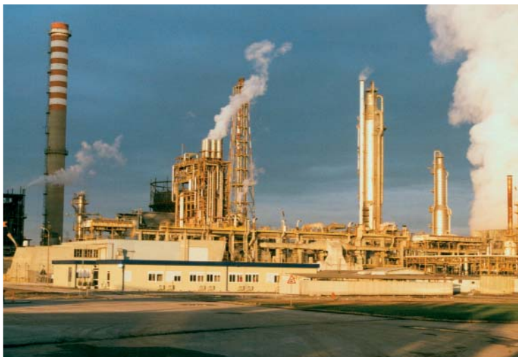
Picture 12. Nitrogen fertilizer plant (Credit: Yara)
