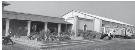
Figure 3. Infrastructure-resource centre (TKVK).
