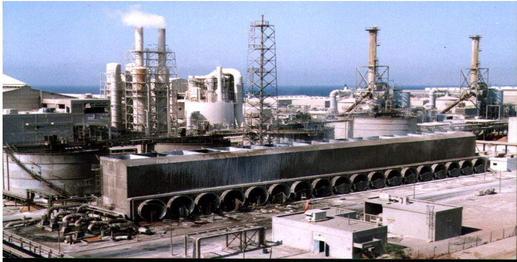
Photo 1. Aqaba Acid Cooling Tower
