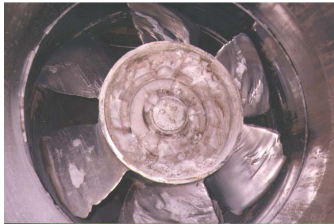
Photo-4. Circulation Axial pump impeller- UB-6 material.
