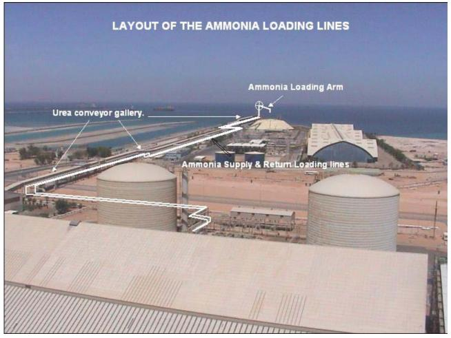
The ammonia plant initially had a rated capacity of 1,000 metric tons per day, which was later increased to 1,050 metric tons per day by incorporating the Hydrogen Recovery Unit.
