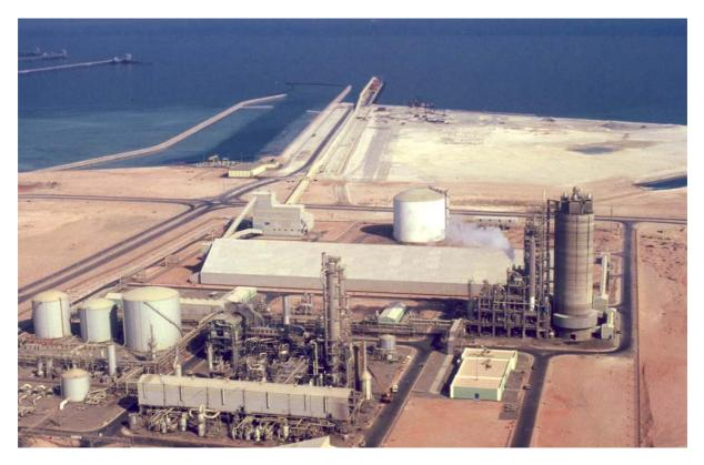
FERTIL's installations are located in the Ruwais Industrial Zone on the Arabian Gulf coast about 240 Km west of Abu Dhabi city. The complex comprises ammonia and urea processing plants with installed capacities of 1050 MTPD and 1500 MTPD respectively. The plants have fully integrated utility units with product handling and shipping facilities. The seawater, desalinated water and power are imported from ADNOC utilities plant.
