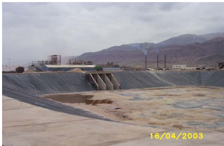
Photo 4: Refinery Collection Pond For Sub-Surface Drainage Water (side view)
