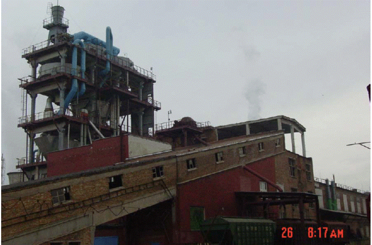
Figure 6: Overall view Grodno granulation with direct loading facility.
