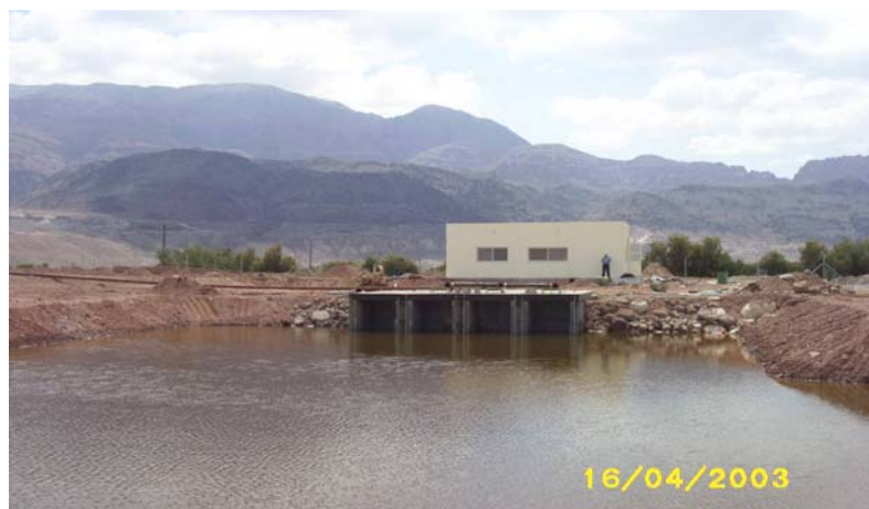
Photo 2: Collection Lagoon For Drainage Water At Sammar Site
