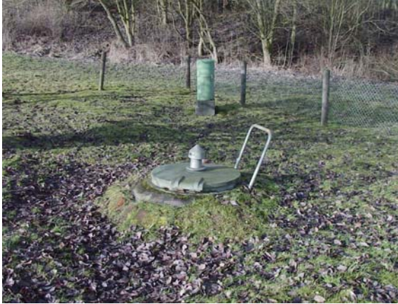
Fig. 5: Groundwater well Ziegelei at Wölfershausen
