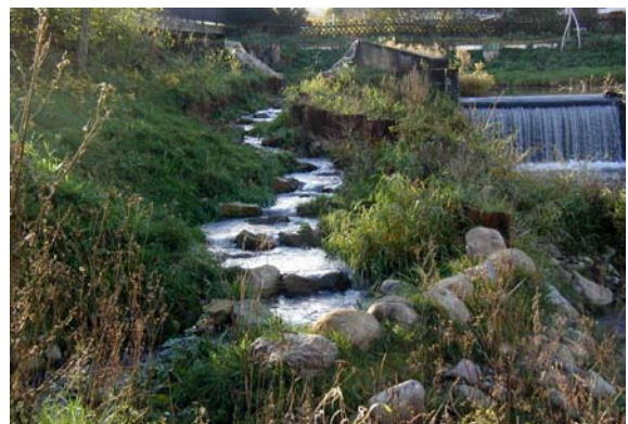
Fig. 2: Fish pass at Salzdetfurth, Lamme river
