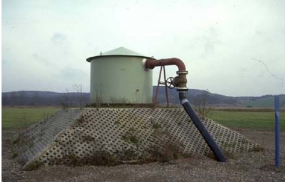
Fig. 7: Deep well disposal of saline water (Herda 10 at Gerstungen)
