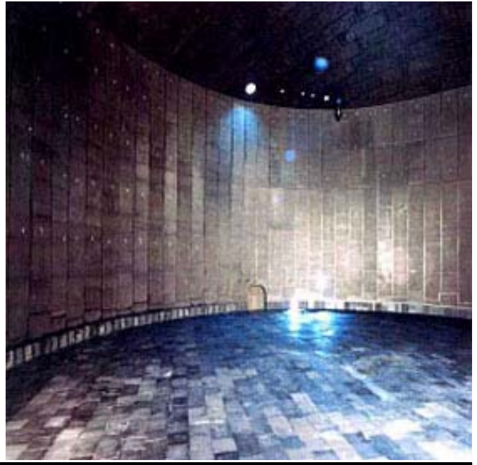
Lining of a storage tank with rubber sheets and carbon bricks
