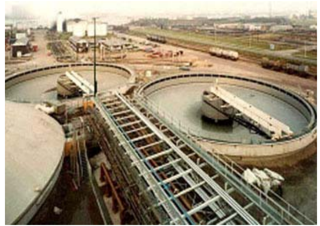
Polymer Lining in Concrete Settling Tanks
