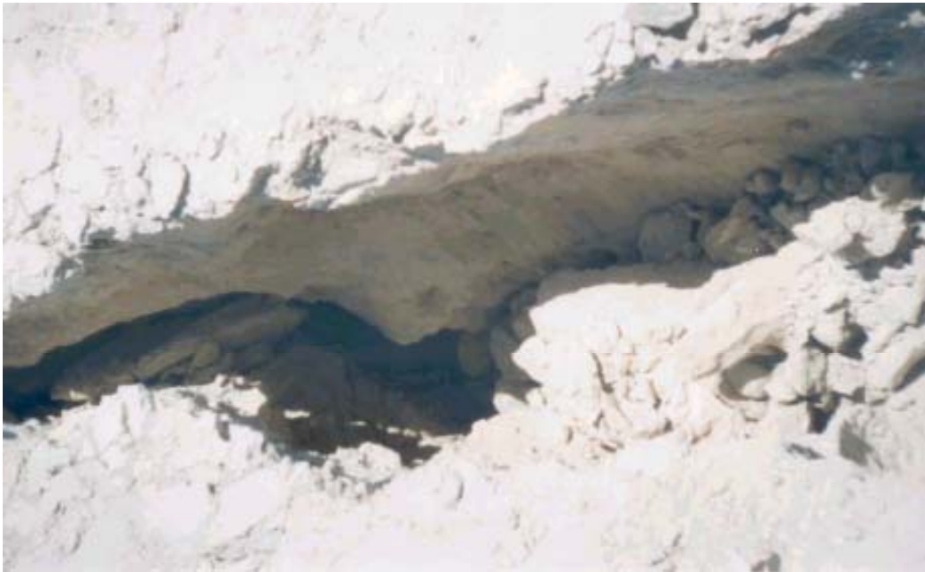
Wide crack near the edge of the stack
