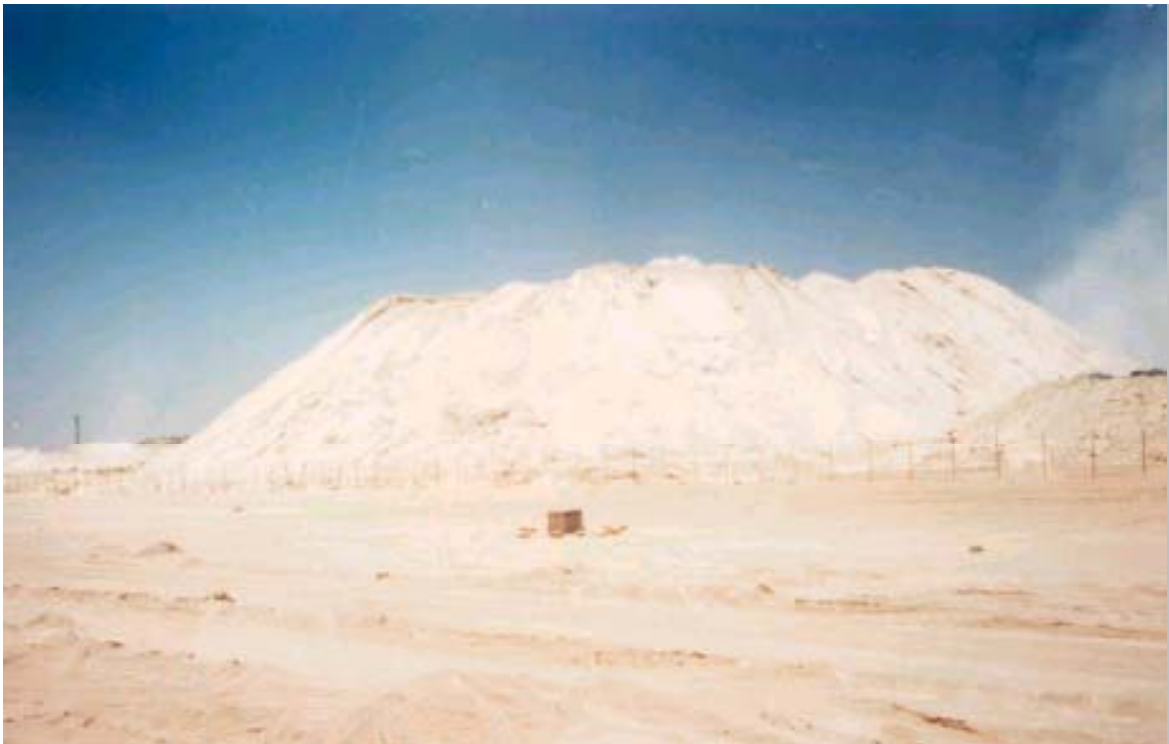
Rear view of the stack at maximum height
