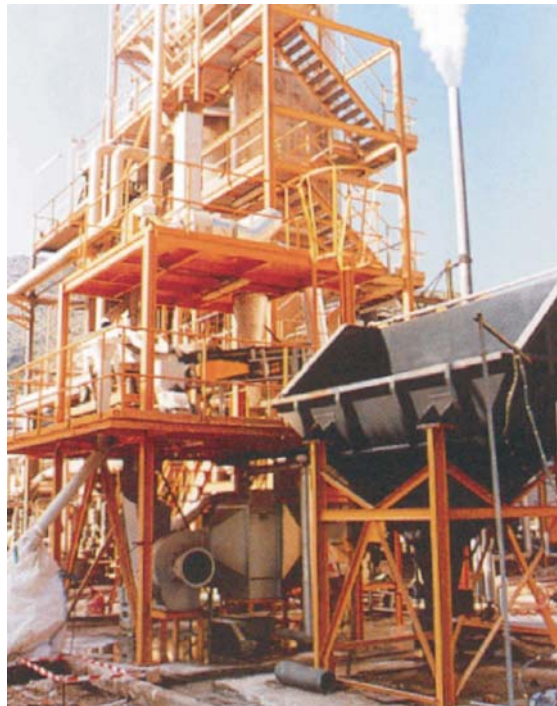
Pilot plant in Fertiberia production facilities
