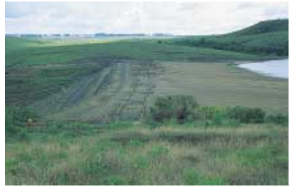
Magnetite tailings dam - Fosfertil, Brazil
