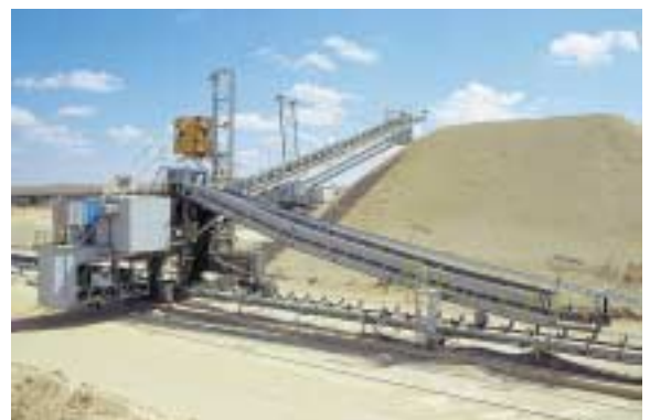
Conveyor and stacker - Office Chérifien des Phosphates (OCP), Khouribga, Morocco
