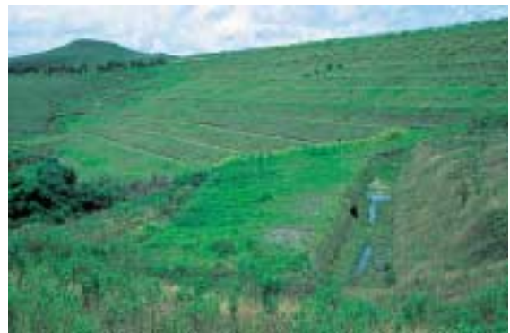
Dam wall, clay fines tailings - Fosfertil, Brazil
