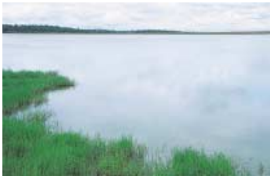
Tailings dam, wall in distance - Copebras S.A., Brazil
