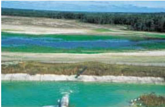
Clay settling pond - Cargill Fertilizers Inc., USA
