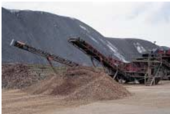
Sorting and crushing demolition rubble - Kali und Salz GmbH, Germany
