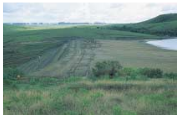
Magnetite tailings dam - Fosfertil, Brazil
