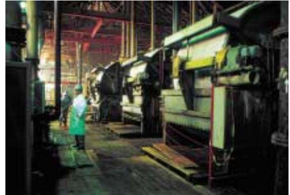
Filtering potash before drying - Kali und Salz GmbH, Germany
