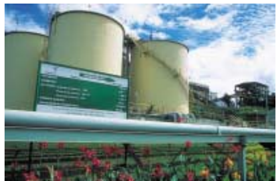
Phosphate rock concentrate slurry tanks and pumping - Fosfertil, Brazil
