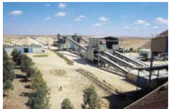
Sizing and stockpile plant - Office Chérifien des Phosphates (OCP), Khouribga, Morocco
