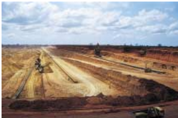
Surface mining of phosphate rock, with bucketwheel - Office Togolais des Phosphates (OTP), Togo
