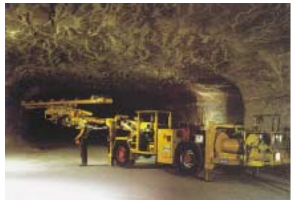
Drilling holes for blasting explosive - Kali und Salz GmbH, Germany
