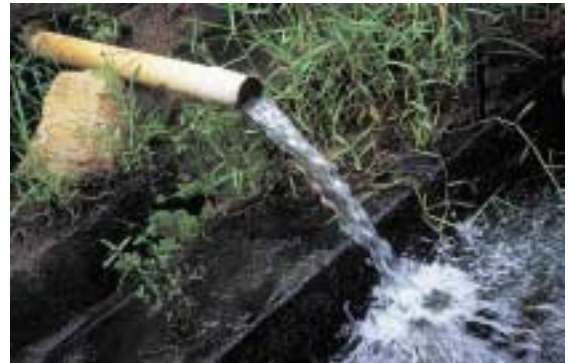
Tailings dam seepage water release - Copebras S.A., Brazil
