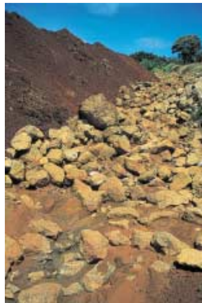
Lined drainage channel - Fosfertil, Brazil
