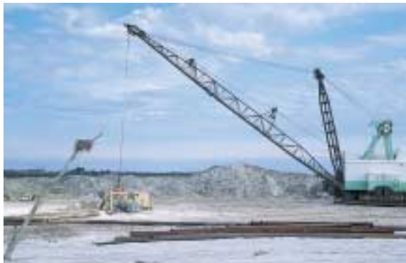
Dragline avoids bird's nest - Cargill Fertilizers Inc., USA
