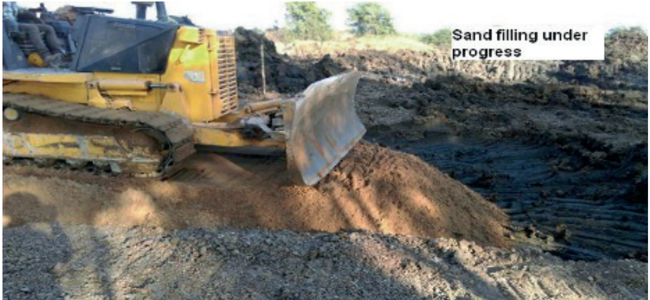
Fig. 111. Application of sand course (Image courtesy Paradeep Phosphate Ltd)
