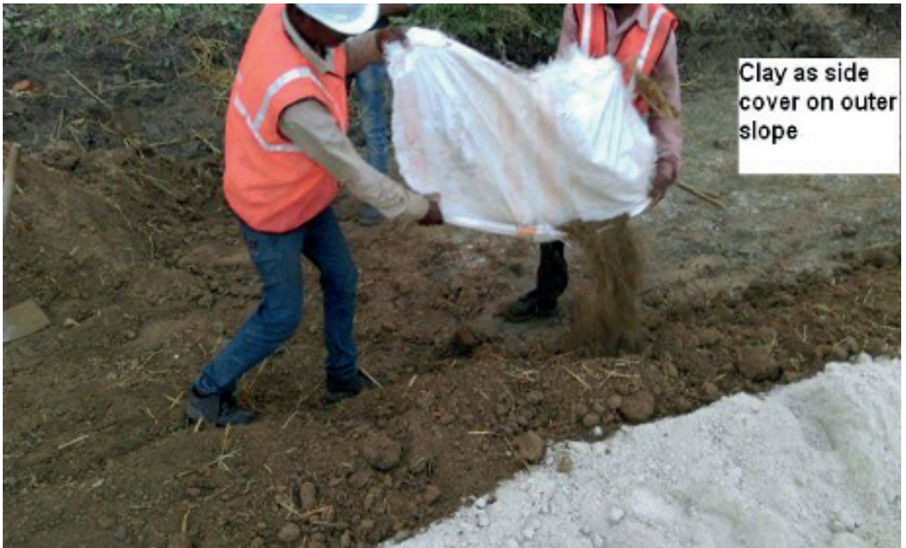
Fig. 113. Clay as side cover, outer slope (Image courtesy Paradeep Phosphate Ltd)
