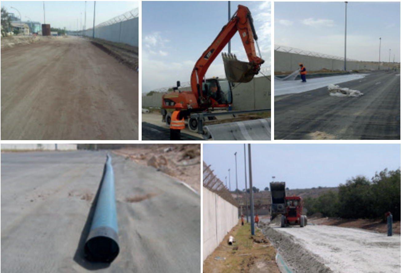
Fig. 105. Road construction with protective impermeable membrane overlaid on Safi naturally occurring soil base course and drainage system for collecting run-off water (Image sequence courtesy OCP)
