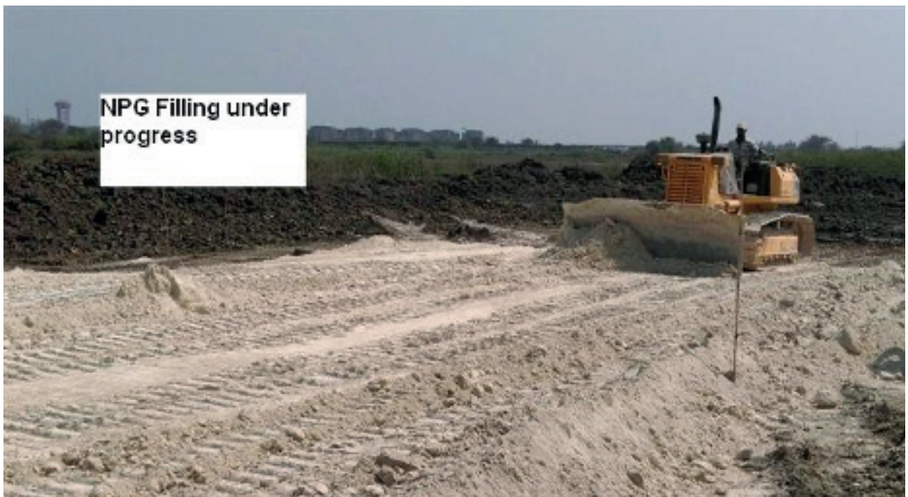
Fig. 112. Development of embankment using neutralised PG (NPG) (Image courtesy Paradeep Phosphate Ltd)
