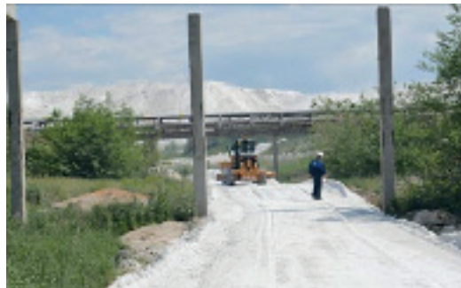
Fig. 93. Leveling off the base course with a land grader (Image courtesy PhosAgro)
