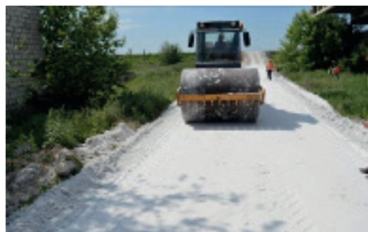
Fig. 94. Light roller compaction (Image courtesy PhosAgro)
