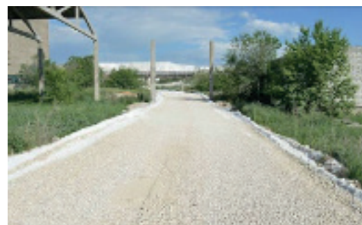
Fig. 96. Condition of the road 24 hours after constructing the base (Image courtesy PhosAgro)
