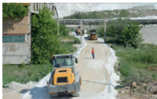
Fig. 95. Spreading and compacting gravel course (Image courtesy PhosAgro)
