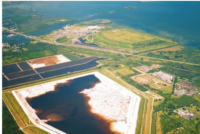
Riverview Existing Stack in Foreground & Closed Stack in Background:
