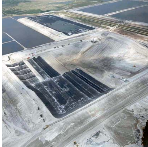
Green Bay Closed Stack Used for Water Storage:
