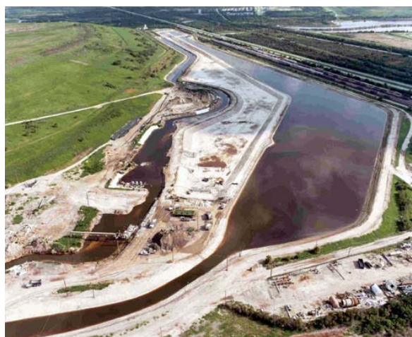
Riverview Process Pond Improvements:
