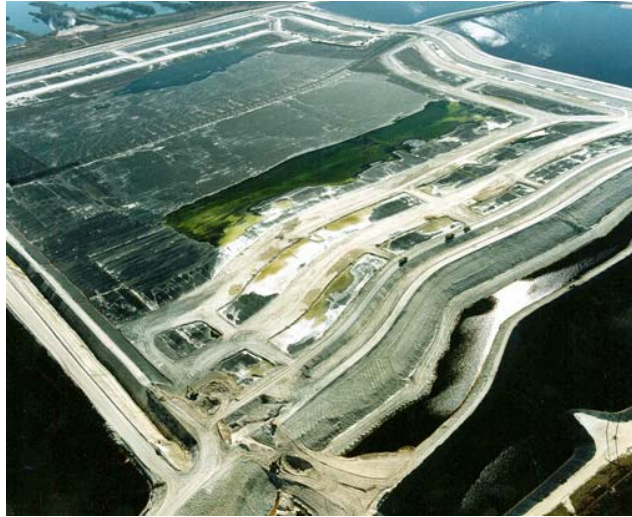
Bartow South Stack Retrofit:
