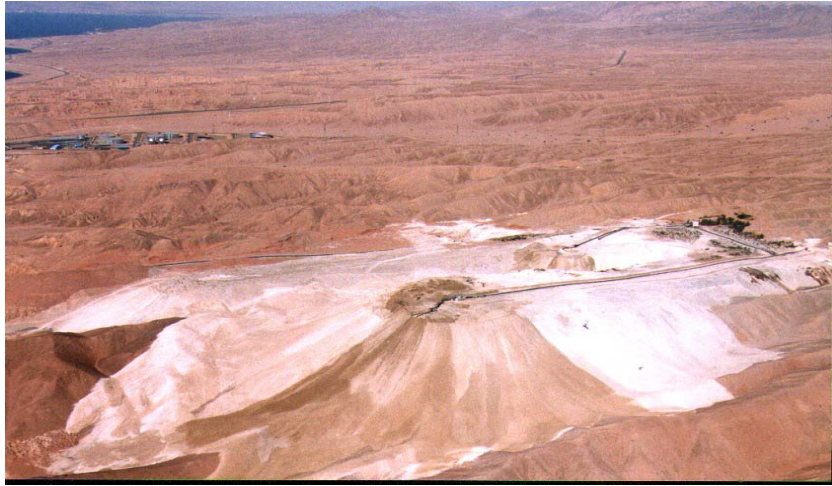
Photo-3. Aqaba Gypsum Disposal & Stacking System.
