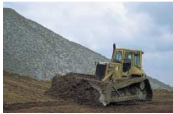
Placing rubble against salt pile - Kali und Salz GmbH, Germany
