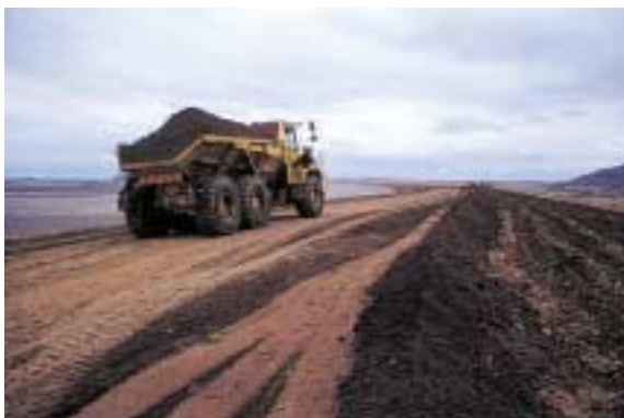
Placing topsoil on dam wall - Foskor Ltd, South Africa
