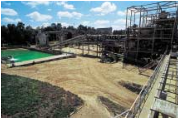
Washing plant - Office Chérifien des Phosphates (OCP), Khouribga, Morocco
