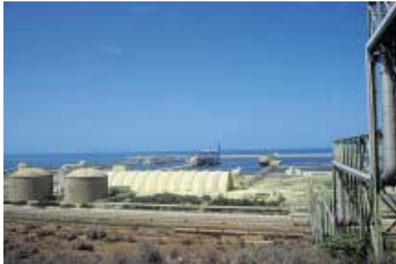
Port, Jorf Lasfar - Office Chérifien des Phosphates (OCP), Morocco
