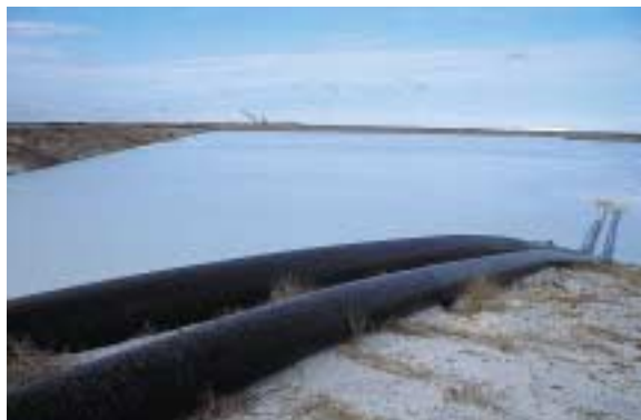
Discharge into clay settling pond (note dragline in background) - Cargill Fertilizers Inc., USA
