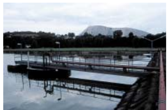
Brine retention ponds for controlled release to Werra River - Kali und Salz GmbH, Germany
