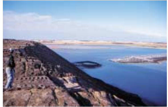
Pond receiving slimes and brine from the stack - Potash Corporation of Saskatchewan (PCS), Canada
