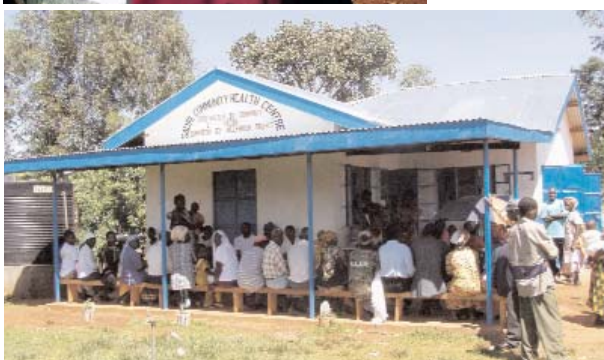
Built by local residents, the new community centre offers free health care to 5000 villagers.
